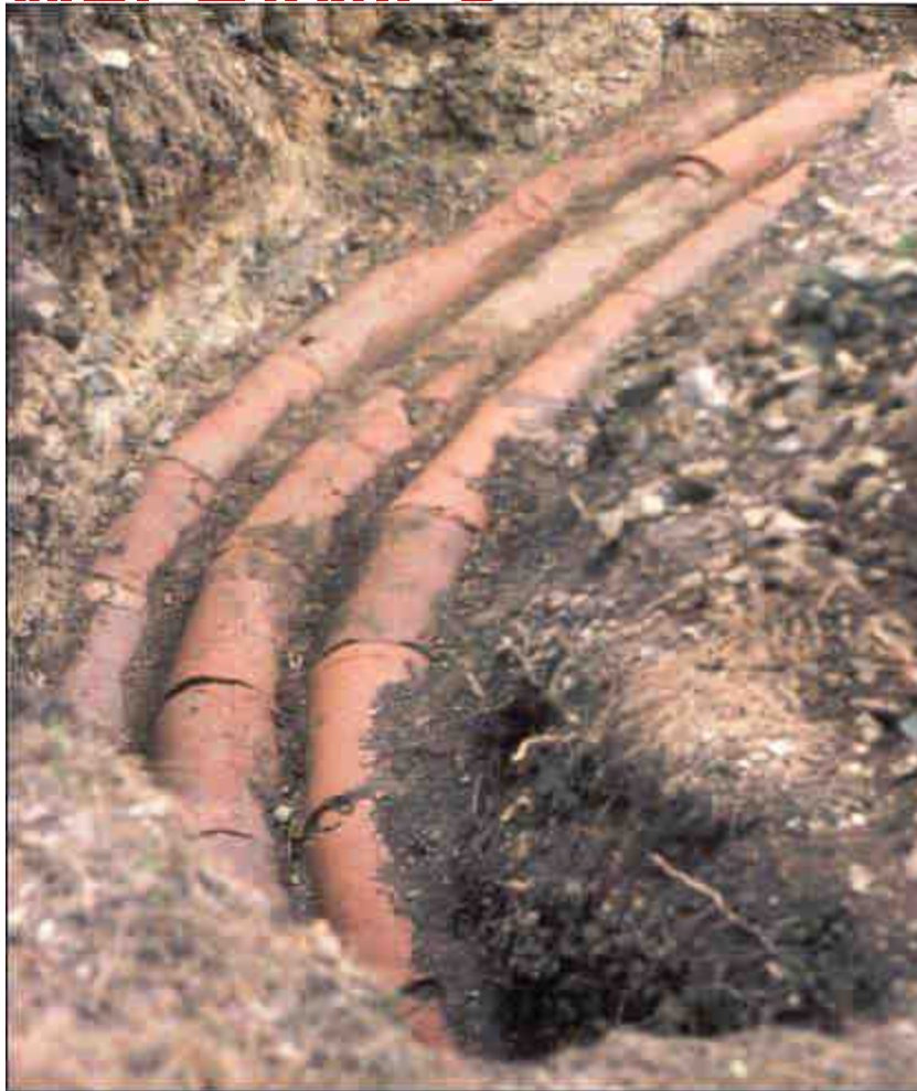
Segment of Pergamon pipeline. Each clay pipe section was 13 to 18 cm in diameter.
