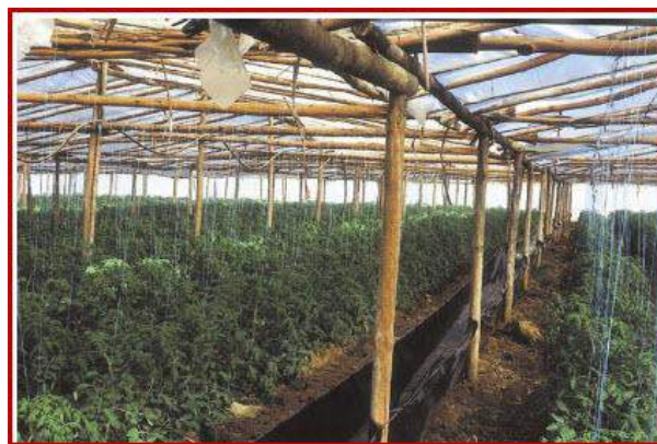
Fig. 1 Wooden framed polyhouse
