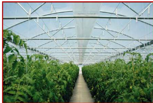
Fig. 2 Polyhouse with steel structure
