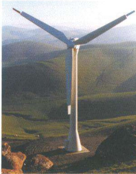
Figure 7.13 A three-bladed horizontal-axis wind turbine (Howden 330 kW)
